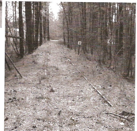
INSPECTING THE OLD LINE
